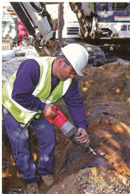
The tank must be opened large enough for a worker to get inside and clean it out. Supervisor Mike Nardone, who also drove the backhoe, makes the cut with a sabersaw while Field Technician Tim Price, below, suits up into protective gear before getting to the heart of the matter, inside the tank.
