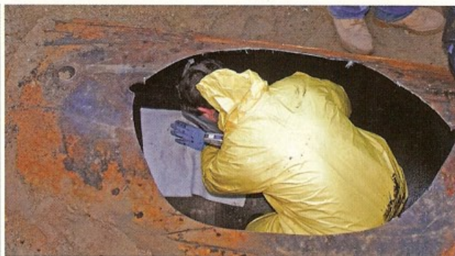
The only way to clean out an old tank is by wiping it out. After having shoveled as much sludge as possible, absorbent wipes pick up the rest of the bottom sediment in this tank. After the cleanup, it will be lifted out (facing page).
