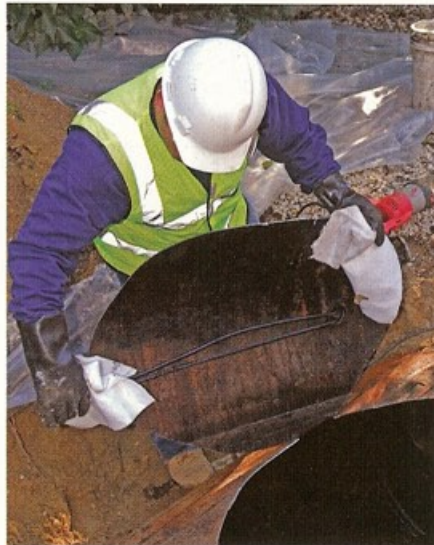
The tank must be opened large enough for a worker to get inside and clean it out. Supervisor Mike Nardone, who also drove the backhoe, makes the cut with a sabersaw while Field Technician Tim Price, below, suits up into protective gear before getting to the heart of the matter, inside the tank.
