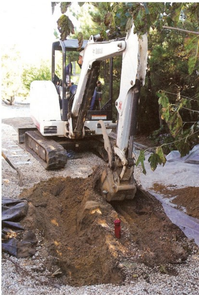
The new tank has been installed, right, and now it's time to dig up the old one.
